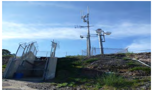
East – Site viewed from the east.
